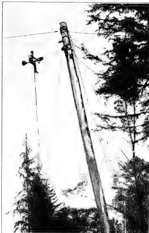
The lumberman calmly smokes his pipe as he oils the blocks at the top of the swaying pole
